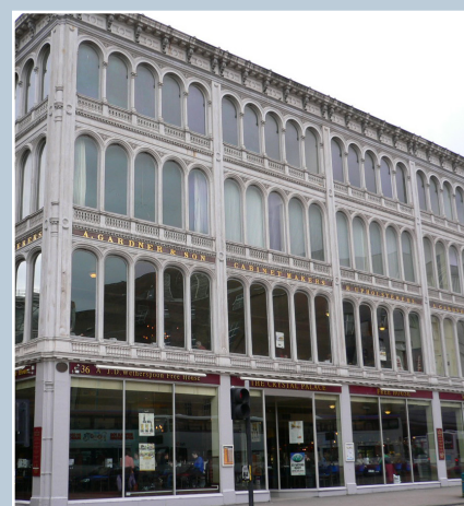
Gardner's Warehouse, Jamaica Street, Glasgow. Now in use as a bar, this pioneering iron-framed building was constructed as a retail warehouse in 1855-6 for A Gardner & Son, cabinet makers and upholsterers. The original lettering was kept at first floor, and new lettering in a similar style fitted to match the new name at the ground floor.
