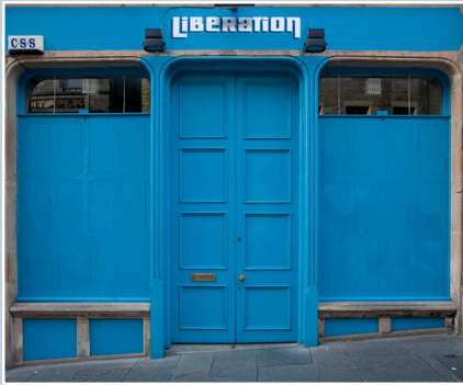
Cockburn Street, Edinburgh. Original later 19th-century timber panelled security shutters that slide down into slots beneath the windows during the day. © N Haynes.
