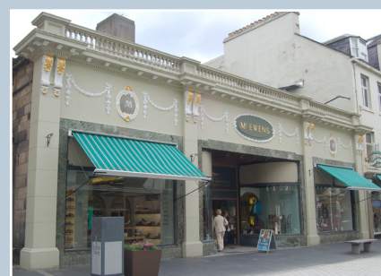
Replacement fabric attached to the traditional awning mechanisms at McEwens, St John Street, Perth.
